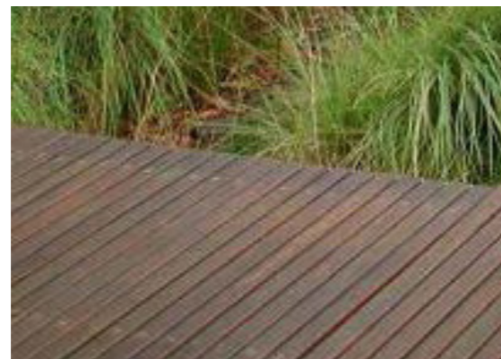
TIMBER DECKING ABOVE SWALE
