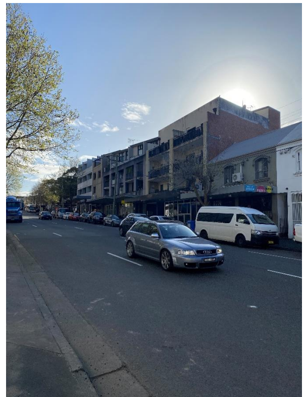
Figure 10 | Development on the east side of Regent Street looking north
